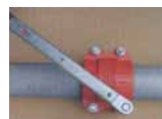
4. Tightening Nuts: Using an appropriate tool, tighten the nuts sequentially until the fittings' housing bolt pads meet, metal to metal.
