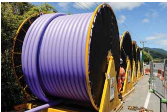
100m Coils – PE telecommunication duct SDR17
