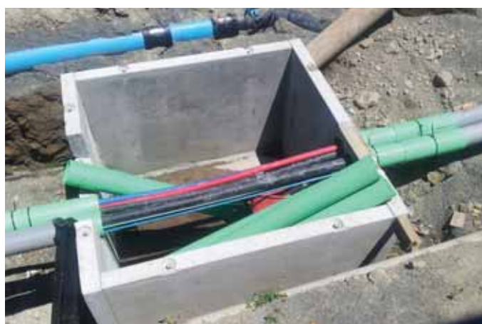
DN 32 PE sub- ducts inside 100mm PVC carrier ducts, at a roadside connection pit
