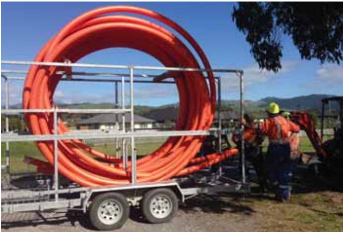
Two DN 110 PE electrical ducts in 50m coils on a dual-coil dispensing trailer
