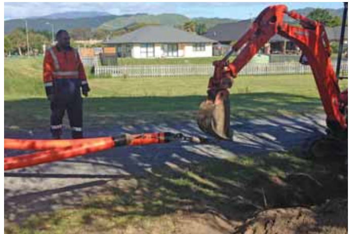
DN 110 PE electrical ducts with pull heads in place, ready for pull-in by horizontal directional drilling
