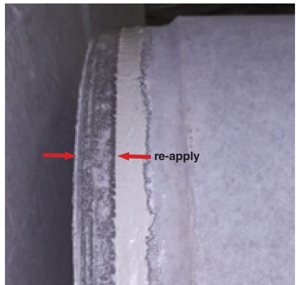
Figure 5. If the pipe needs to be re-connection during this process, re-apply lubricant to ensure smooth installation.
