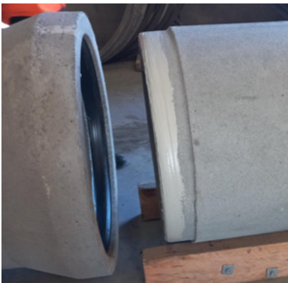
Figure 4. Lower the pipe carefully, ensuring the spigot end is aligned with the collar lip of the receiving pipe before homing together.
