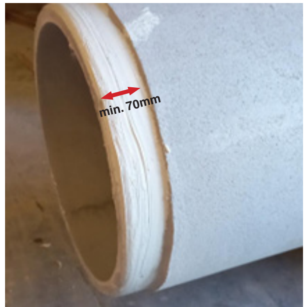
Figure 3. Ensure the spigot edge is fully coated with lubricant and has a min. 70mm coverage on the entire spigot surface circumference.
