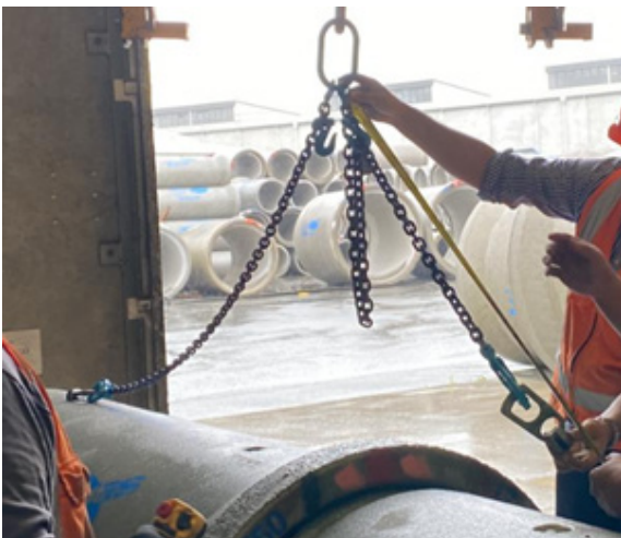
Figure 7. Long chain on the far side of the lifting pin on the receiving pipe, the short chain connected to the closer side of the pin of the homing pipe.
