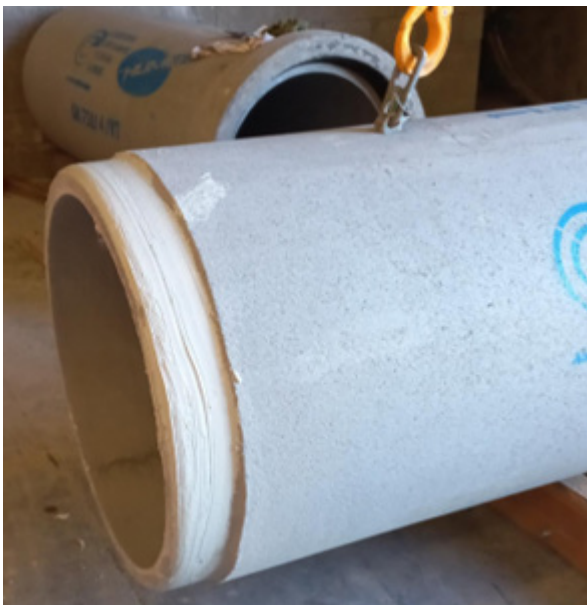
Figure 2. Wearing protective gloves, apply lubricant on the Spigot area; do not apply with a brush.
