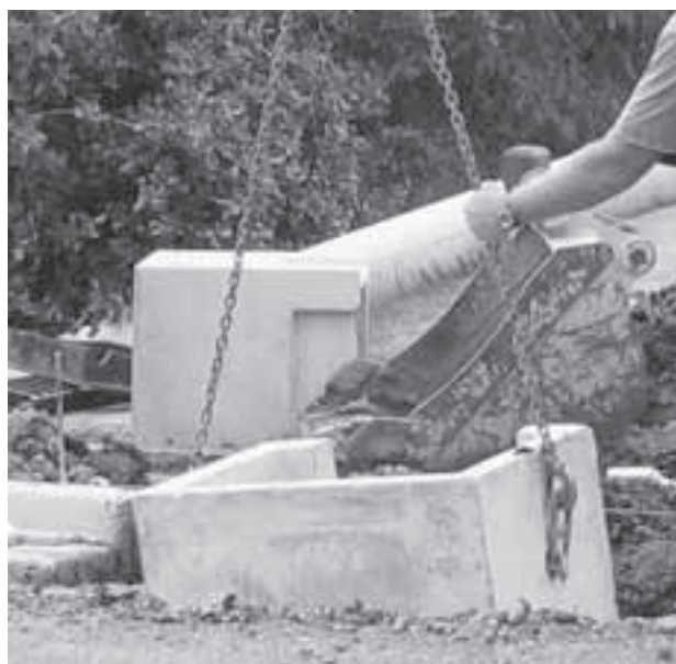
Cesspit installation
