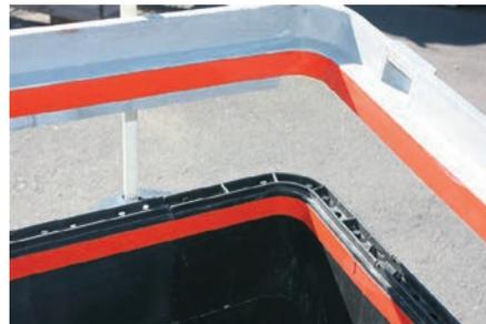
3. Cut four corner pieces from roll of shuttering material approx 30cm long.
