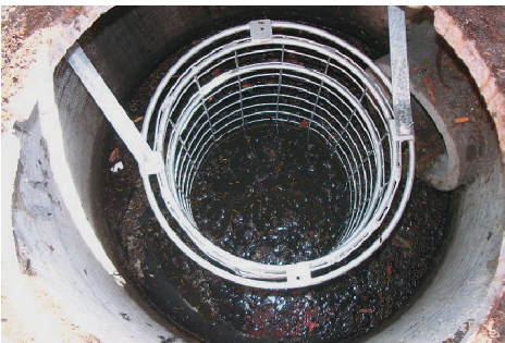
Curb Inlet Manhole Enviropod®
