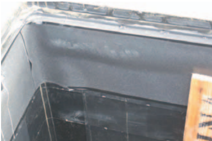
1. Shuttering system correctly installed
