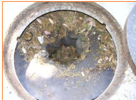
Curb Entry Manhole EnviroPod
