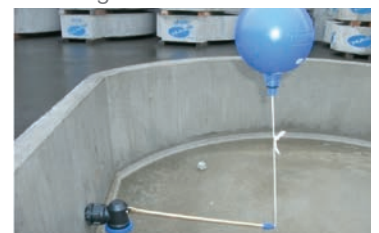
Inlet for all CT Troughs Please Note: No protection for valve and float.
