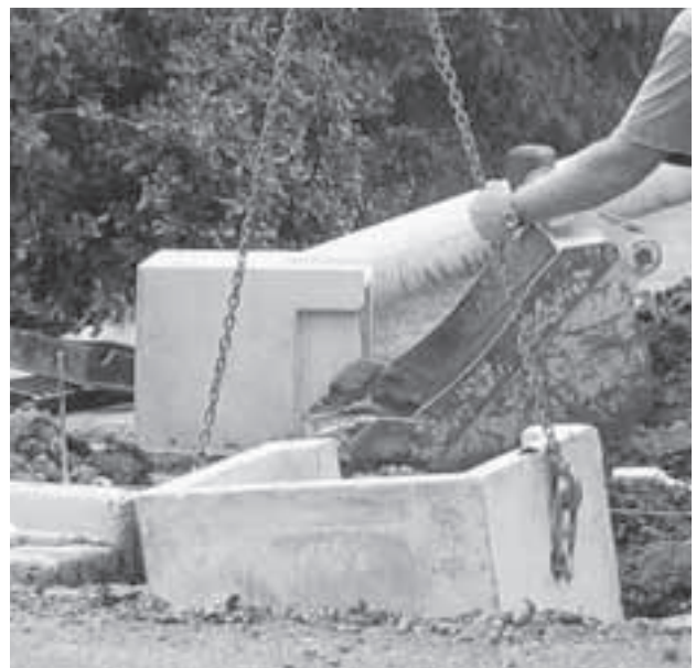
Cesspit installation
