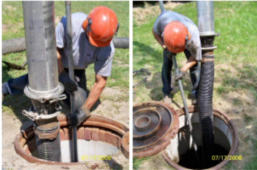
A maintenance worker stationed on the surface uses a vacuum hose to evacuate water, sediment, and debris from the system.
