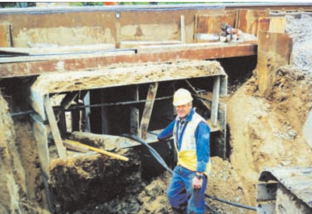
Top: The custom designed boxes on site ready for installation.
