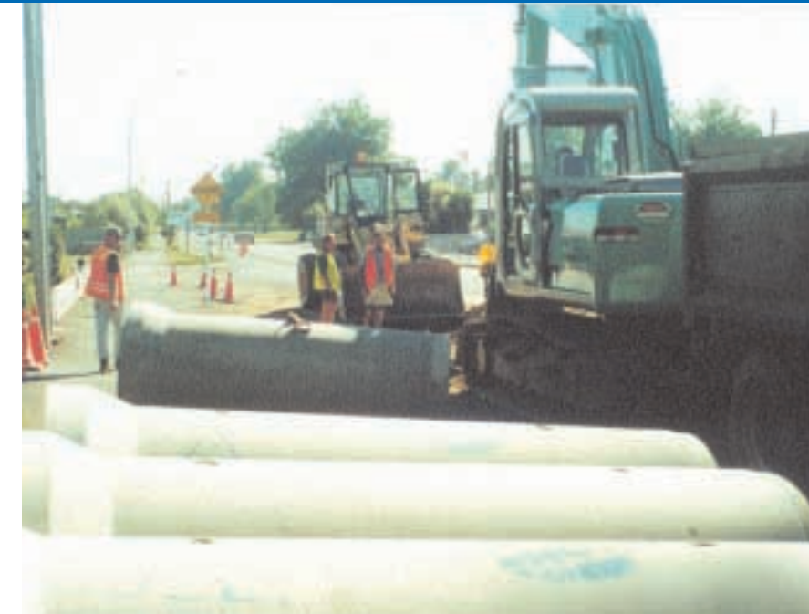
Left: Special handling was required for the Duracem manufactured pipes.
