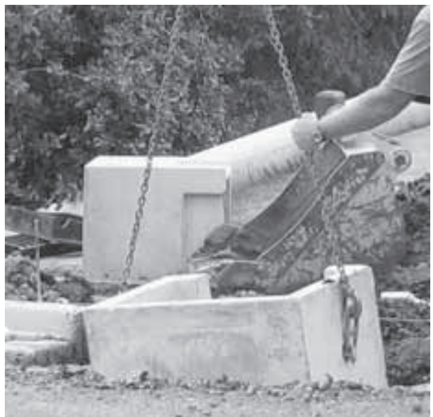
Cesspit installation
