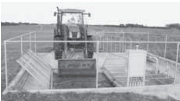
Stone trap incorporated into a Humes Effluent Management System (Refer the Humes Effluent Management System brochure for more detail)
