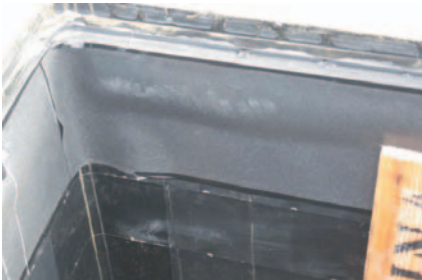
1. Shuttering system correctly installed
