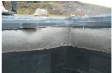
2. Correct concrete finish
