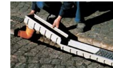
Installation of outlet or sump.
