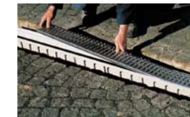
Channel with grate across joint and concrete at joint.
