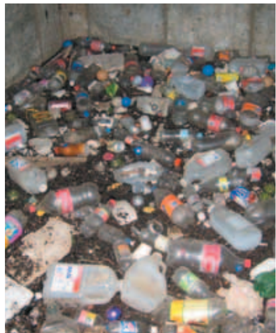
Rubbish and debris captured and retained inside a Humegard™ unit
