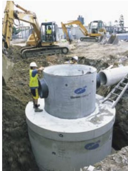
STC18 Humeceptor™ ready for back filling and pipe connection. Note Kor-N-Seal® boots ready to accommodate inlet/outlet pipes.
