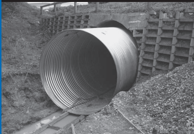
Lightweight and strong large diameter culvert option.
