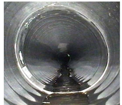
Deflected flexible pipe profile
