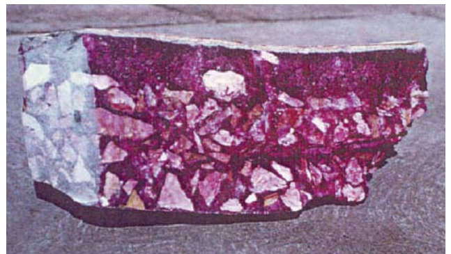
Progress of carbonation in 65 year old spun concrete pipe, exposed to weather. The pink phenolphthalein displays where there is NO presence of carbonation.
